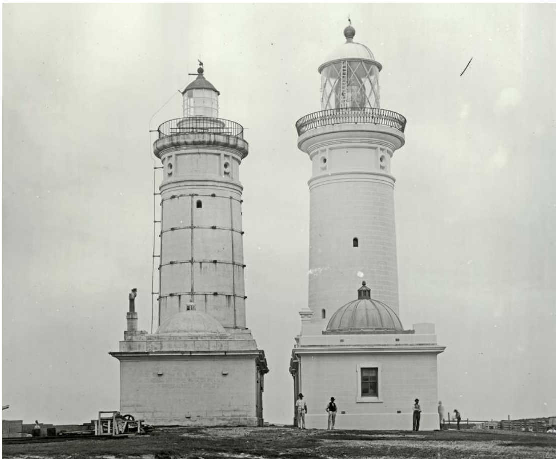
Greenway's and Barnet's Macquarie Lighthouses side by side
