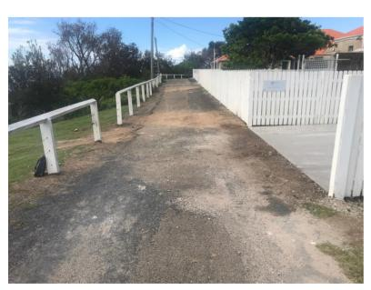
Recent heavy rains and construction activities have resulted in a complete failure of the pavement along the rear access road.
