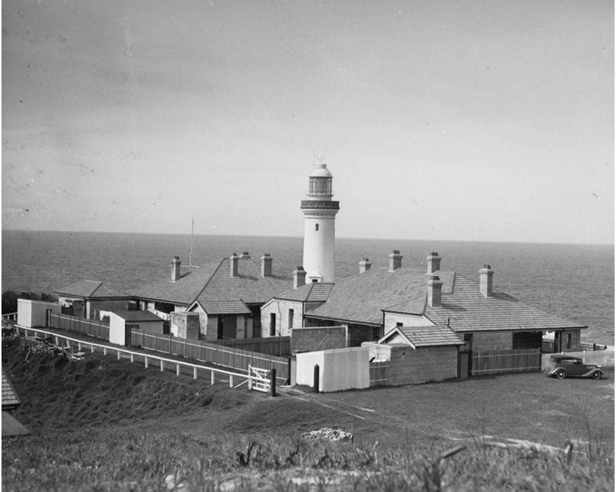
The Quarters are constructed out of concrete blocks cast on site in 1902. They have been cement rendered and pointed to give the appearance of sawn stone. One chimney in Quarters Q3 was not demolished but is not believed to be at its original height.
